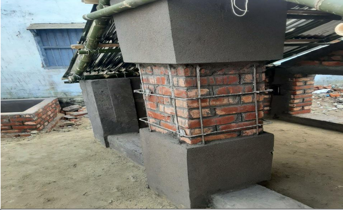
Mason Training on 15-21 January 2021 at Madhepura District
